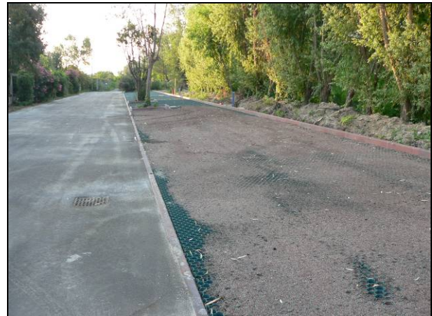
Fig. 2 Installation of the grids
