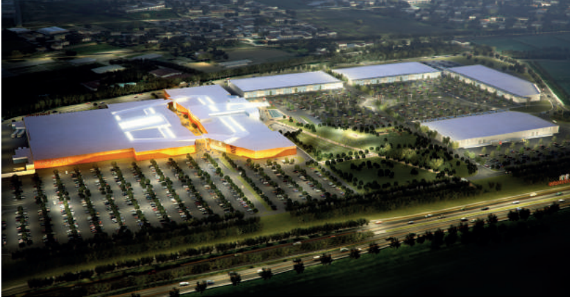
ELEVATOR TANK MondoJuve shopping mall TORINO, ITALY
