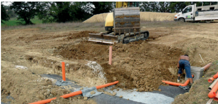
⑤ LAYING OF GETOTEXTILE Lay geotextile over the whole surface.
