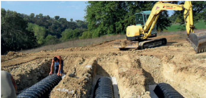
③ INSTALLATION OF DRENING Install the Drening chambers
