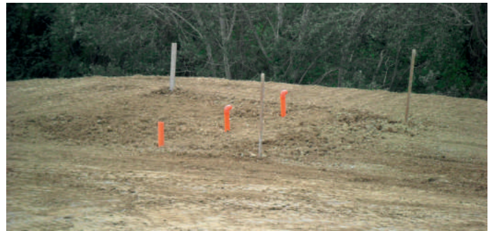
⑥ COMPLETE FILLING Cover until the ground level has been reached.
