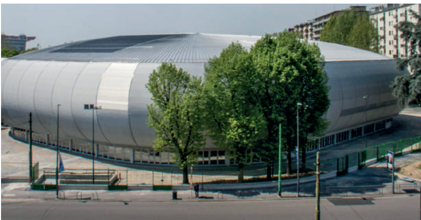
DRAINPANEL Allianz Cloud Sport Hall MILANO, ITALIA
