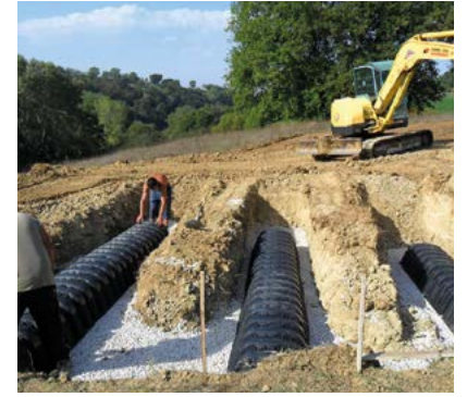
③ INSTALLATION Pose des chambres DRENING.
