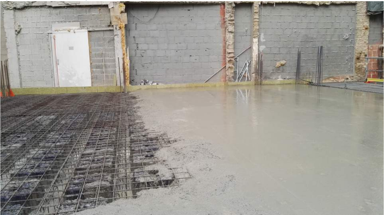
Figure 14 - Cast of the completion layer
