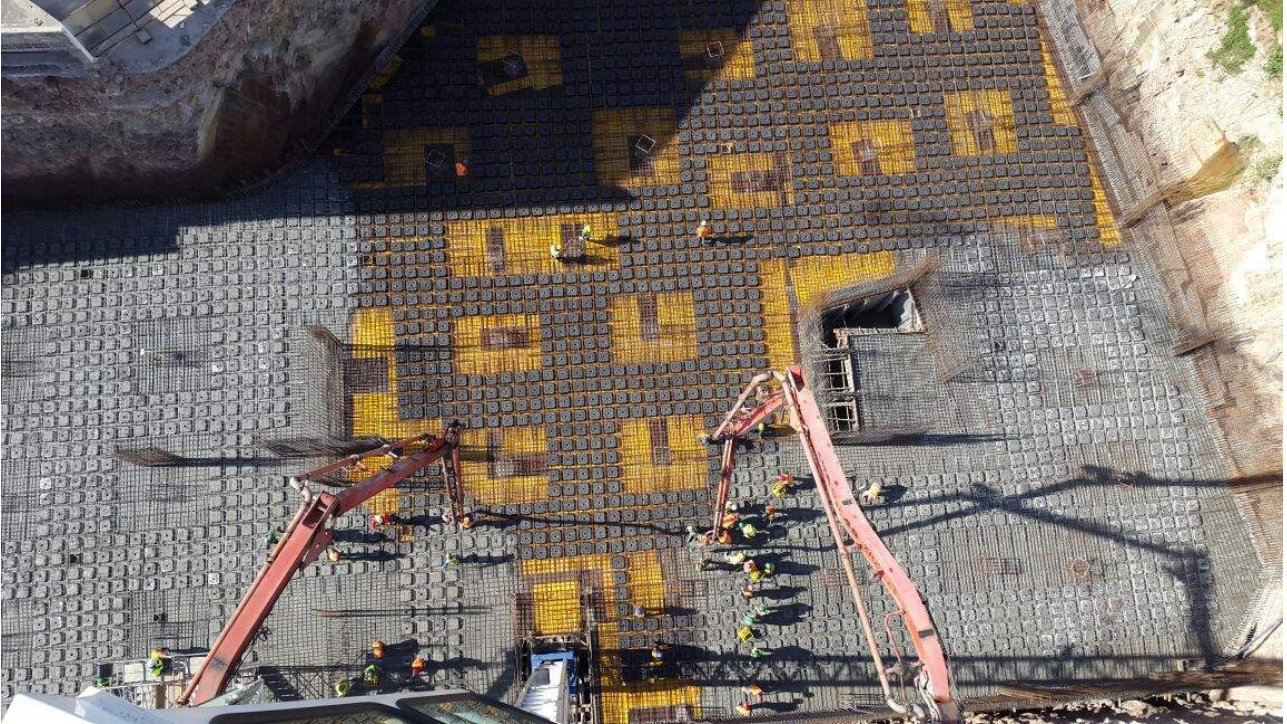
Figure 13 - Cast of the first layer
