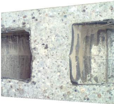
Figura 4 -A section of lightened slab with "double"elements
