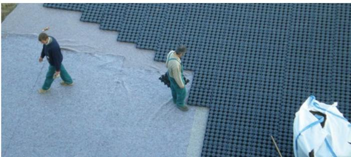
Figura 11 - Posa in opera Drainroof
