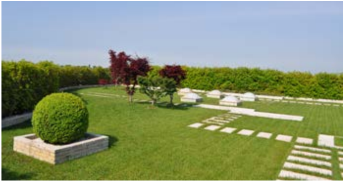
Figure 27 – Example of an intensive roof garden
