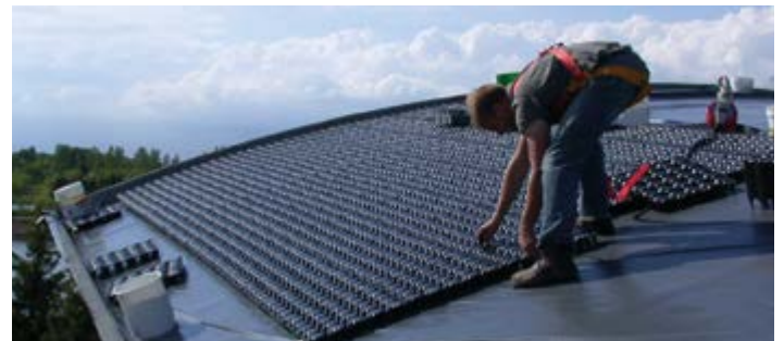
Figure 12 - Drainroof Installation
