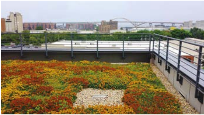
Figure 22 -Example of extensive roof garden on an industrial building
