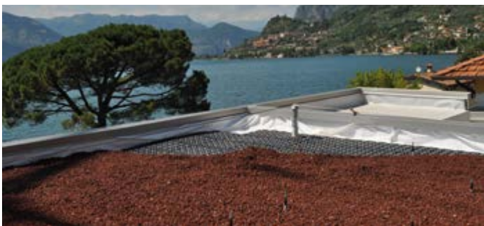
Figure 20 - Combined use of Drainroof and the volcanic lapillus
