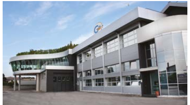
Figure 6 - Geoplast Spa Headquarters
