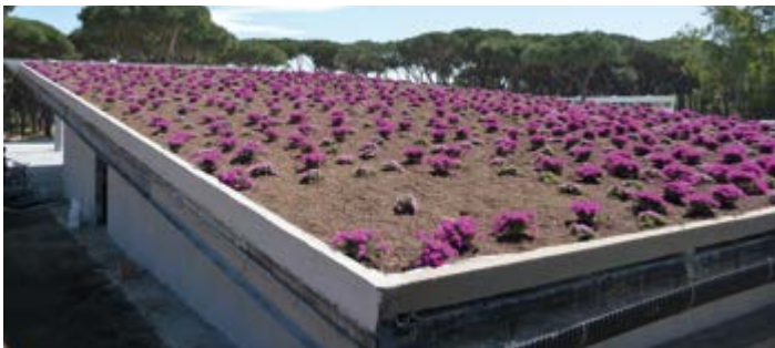
Figure 10 - Installation on curve surfaces
