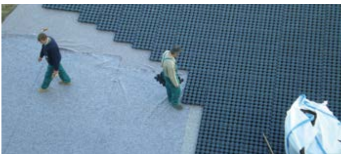
Figure 11 - Drainroof, on-site installation
