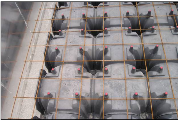
Fig. 1 Biomodulo installed and ready for the pour
