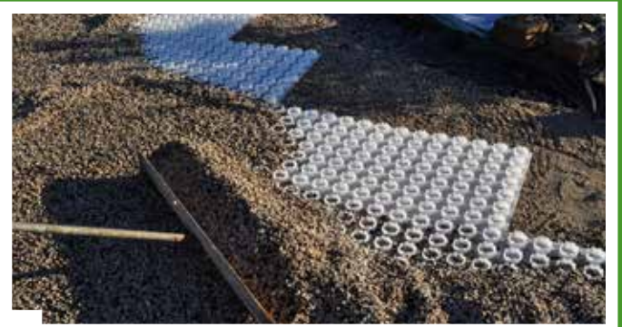
FILL THE GRID WITH FINE PEBBLE FROM 0-5 MM UP TO 3 CM ON THE CELLS
