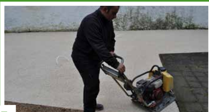
GRAVEL MANUAL COMPACTION
