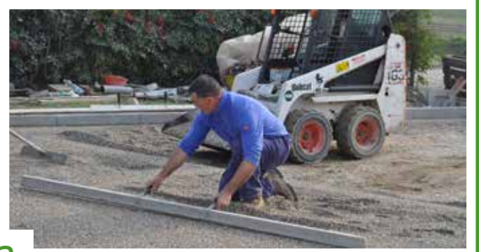
INSTALLATION OF A FINE PEBBLE LEVELLING LAYER 0-5 MM
