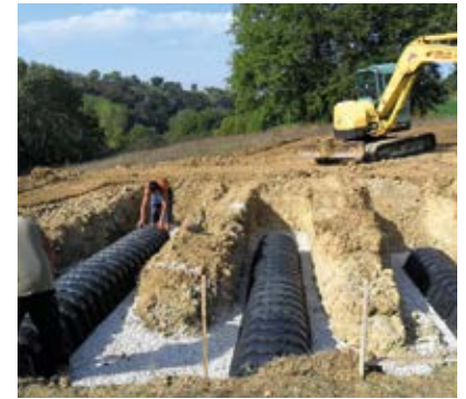
③ DRENING Installation of DRENING chambers.
