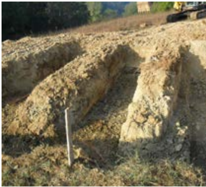
① EXCAVATION Excavation of a dugout 90 cm wide at the base.
