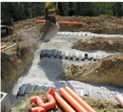
④ COVERING Insertion of the supply and ventilation pipes. Cover with min. 15-20 cm of gravel 20/40 mm.
