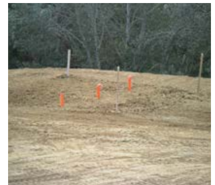
⑥ BACKFILL Backfill until reaching the ground level.
