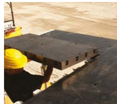
③ POSA PANNELLI GEOPANEL
