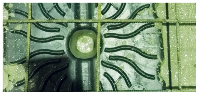
Figure 55 - cone correctly filled
