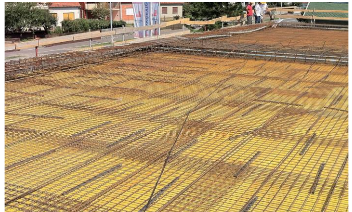
Figure 41 – laying of the lower reinforcement mesh
