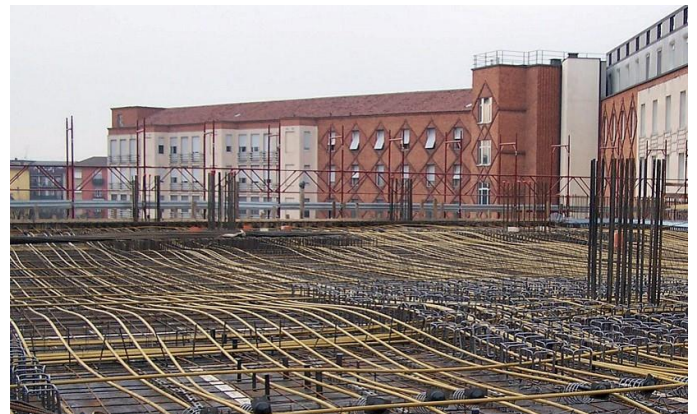
Figure 64 - post-tension cables on plate slab
