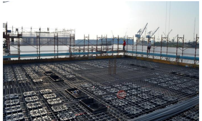
Figure 50 - laying of the upper reinforcement bars
