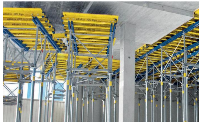
Figure 40 - formwork of cast-in-situ slab with modular wooden formworks
