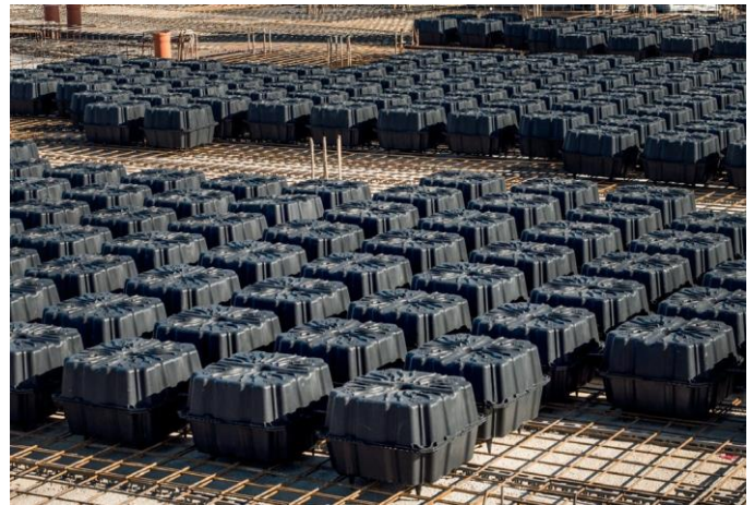
Figure 3 – layout of lightening New Nautilus Evo double
