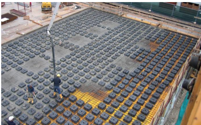
Figure 58 - casting of the first layer
