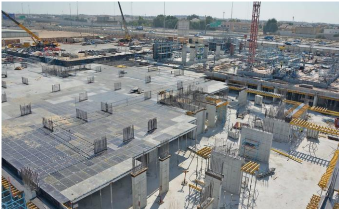
Figure 38 - formwork of cast-in-situ slab with modular metal formworks
