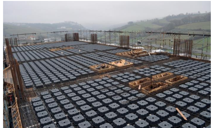
Figure 59 - preparation of cavities before casting
