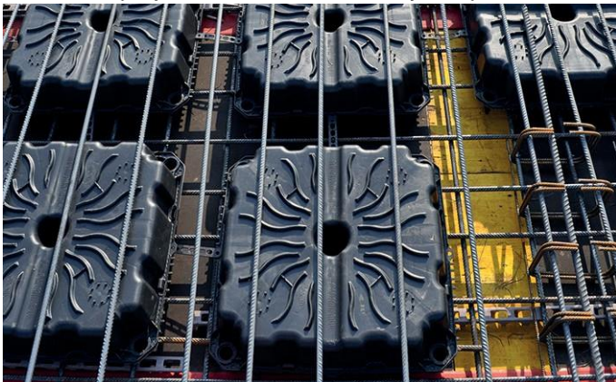
Figure 49 – placing of the upper reinforcement bars
