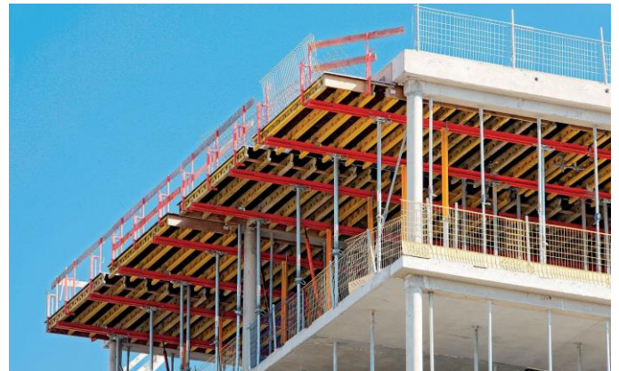
Figure 39 - formwork of cast-in-situ slab with traditional wooden formwork and plywood panels
