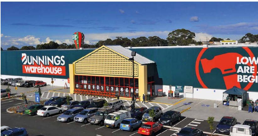
Bunnings Warehouse SYDNEY, AUSTRALIA
