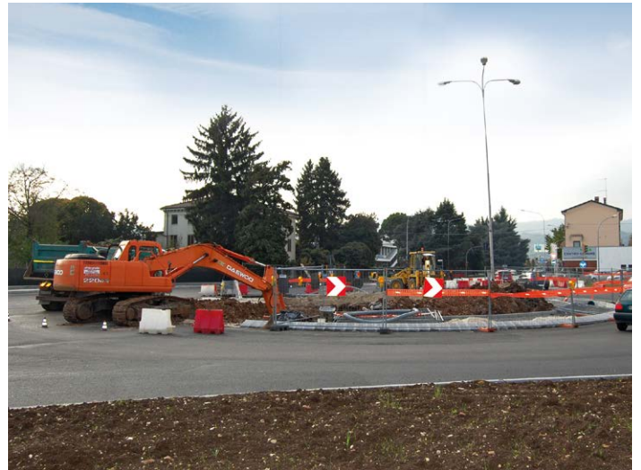
⑤ Final work of kerb repositioning and planting of plants.
