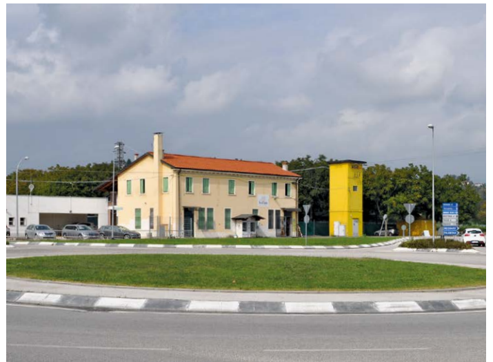
⑥ Completed roundabout.
