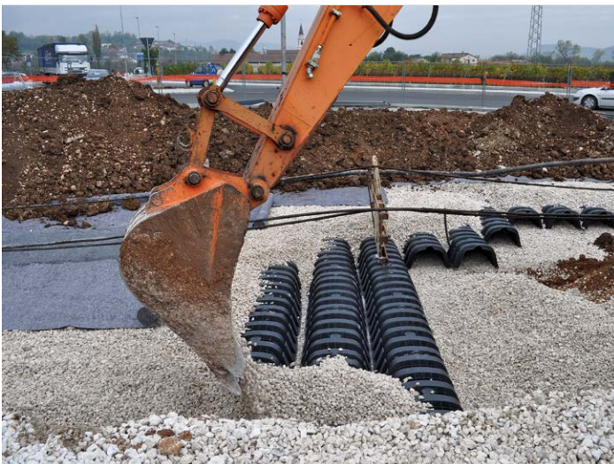
③ Covering of the drainage modules with gravel.
