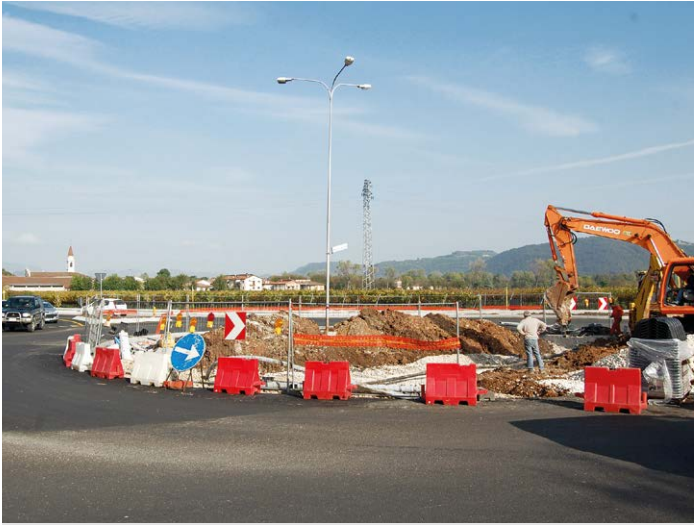
① Excavation and splatting works.
