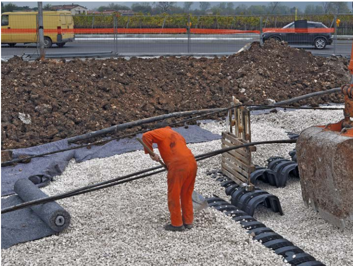
② Installation of gravel bed, geotextile and Draining modules.
