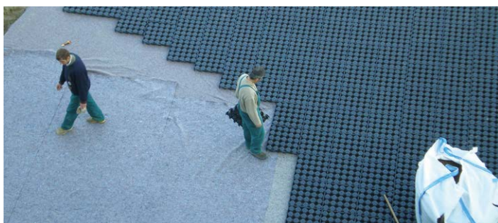
Figura 11 - Posa in opera Drainroof
