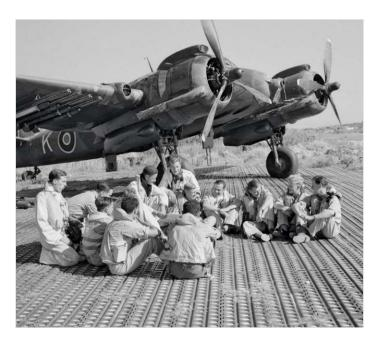
During the Second World War the allies developed a system of perforated and modular steel grids, called "Marston Mats", which stretched on the ground and united to others were used for the rapid preparation of airports and roads. The Italians called them "perforated metal grids", neologism derived from the English term "grill" that means grid.
