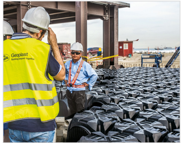
Modulo on-site installation
